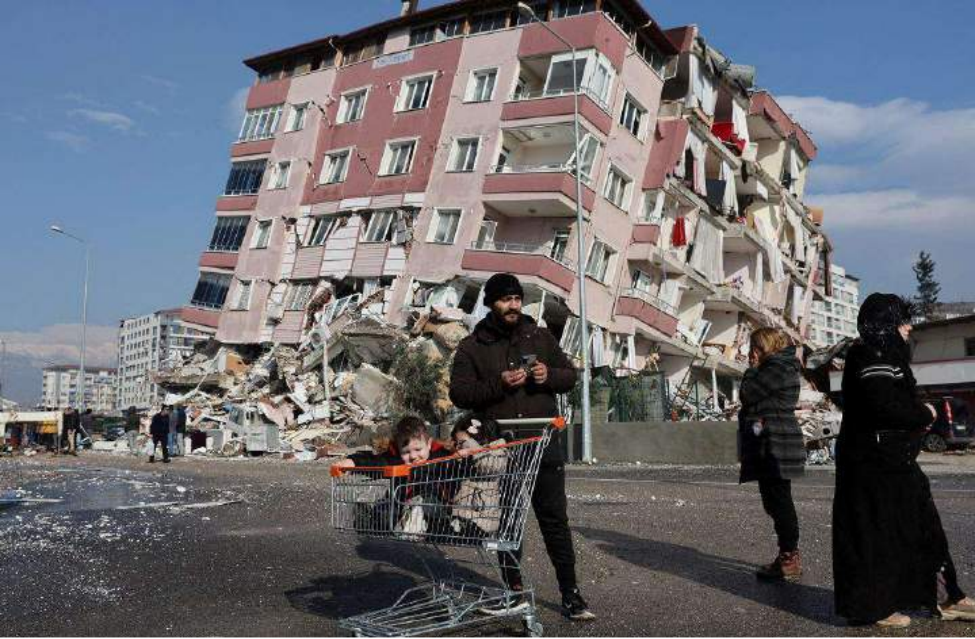
A collapsed building in Hatay, Turkey, February 7, 2023. (Photo: REUTERS/ Umit Bektas/ File Photo)
