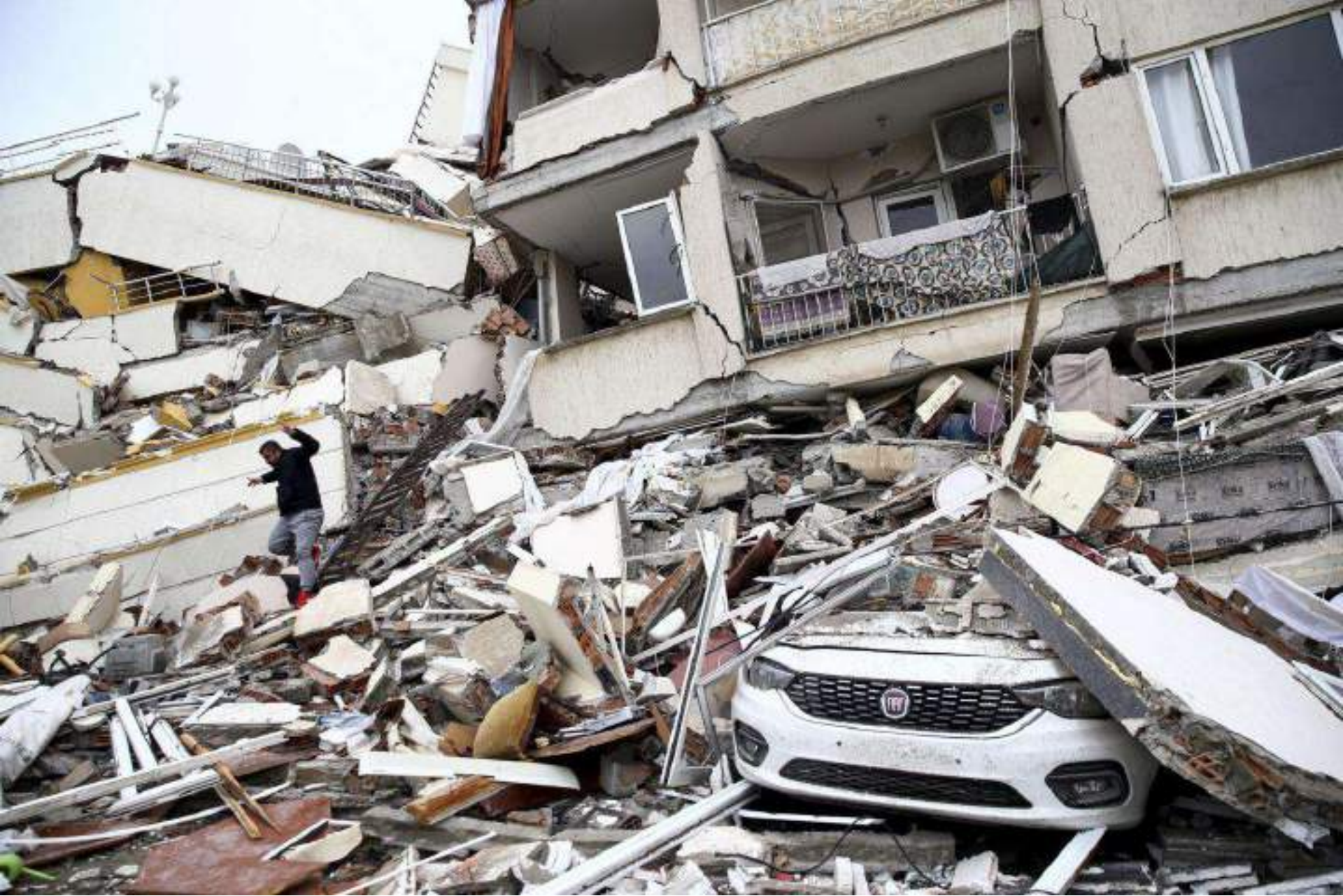
Rubble of a collapsed building in Hatay. Sezgin Pancar/Anadolu Agency/Getty Images
