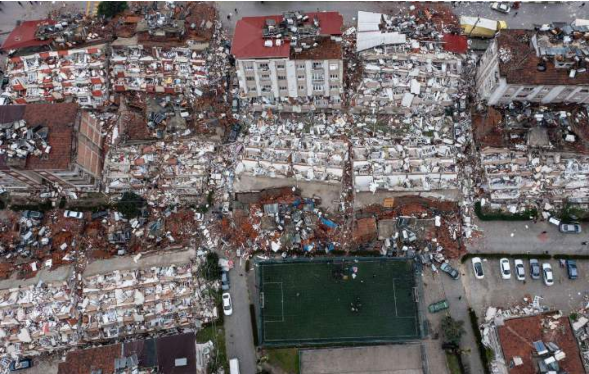
Flattened buildings in Hatay Credit: Anadolu Agency, Erçin Ertürk
